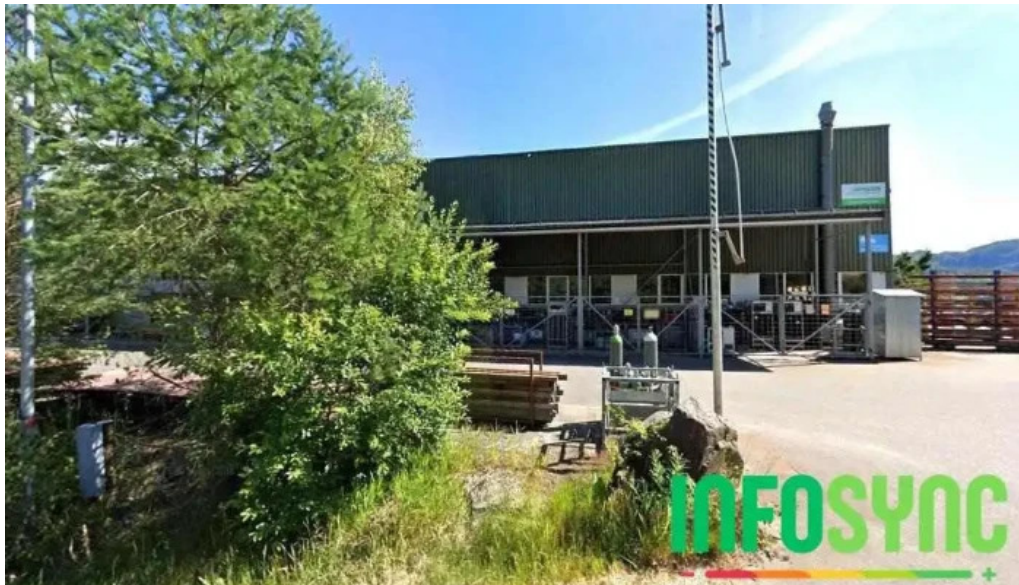
Agder tunnelservice as terox group as flekkefjord
