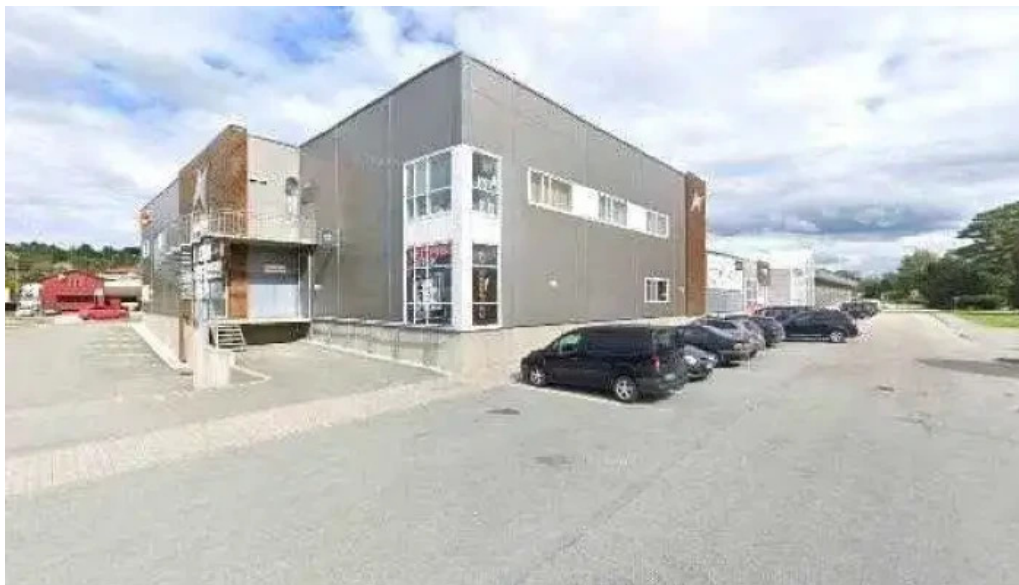
Sunwind hyttesenter rissa street view 360deg
