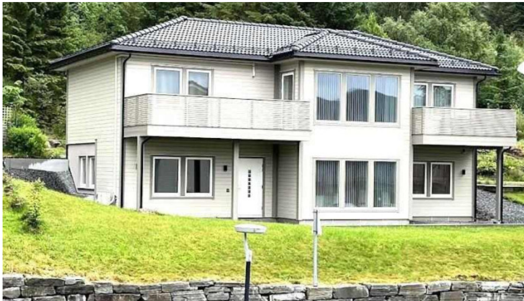
Solund bygg as hardbakke
