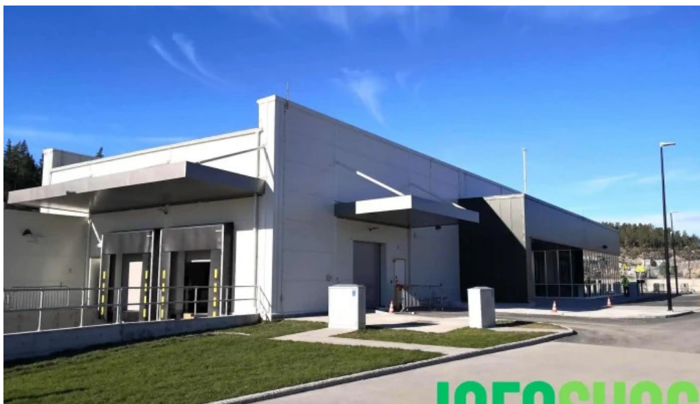
Green mountain dc3 ytre enebakk alle
