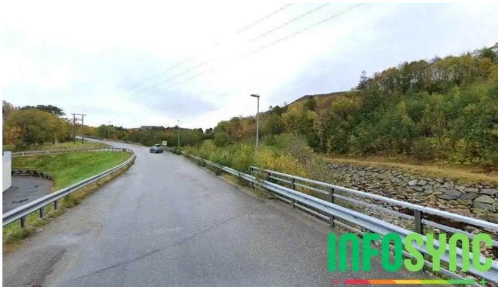
Lauvsnes power station flatanger
