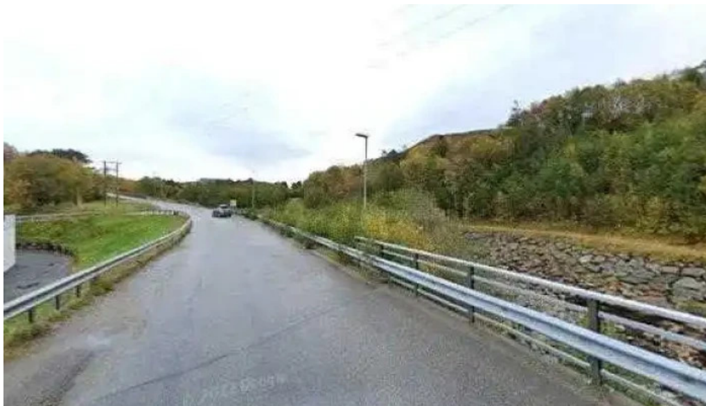
Lauvsnes power station alle
