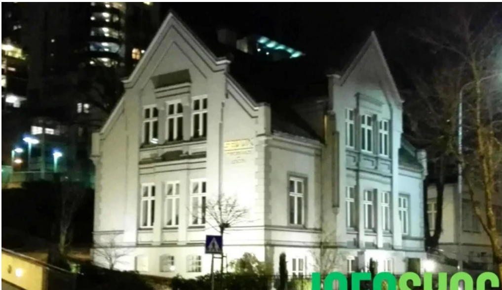
Rebuild as eksterior
