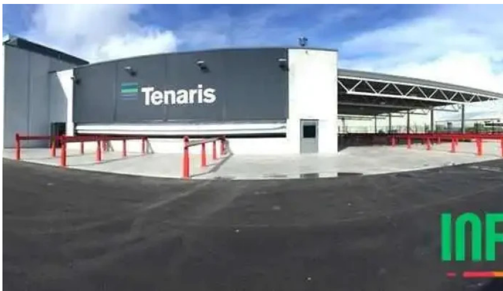
Tenaris global services norway as inspection facility tananger tananger
