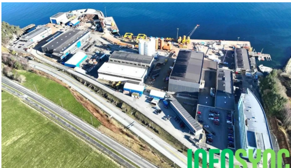
Randaberg industries as bygning
