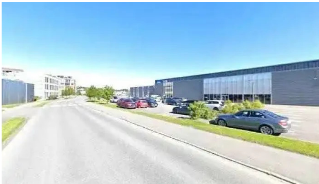
Caverion levanger street view 360deg
