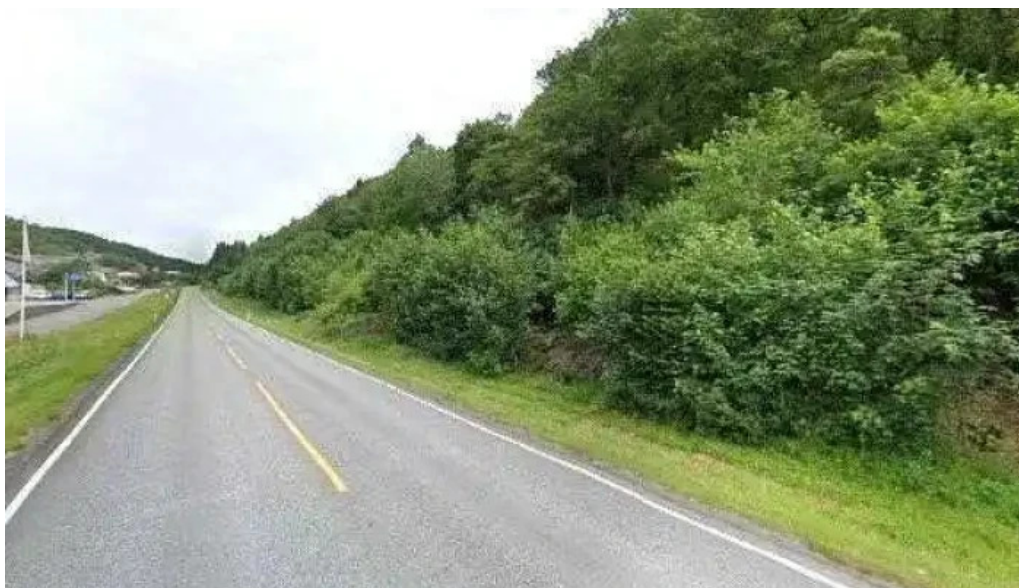
Skaland rør industrimontasje as street view 360deg
